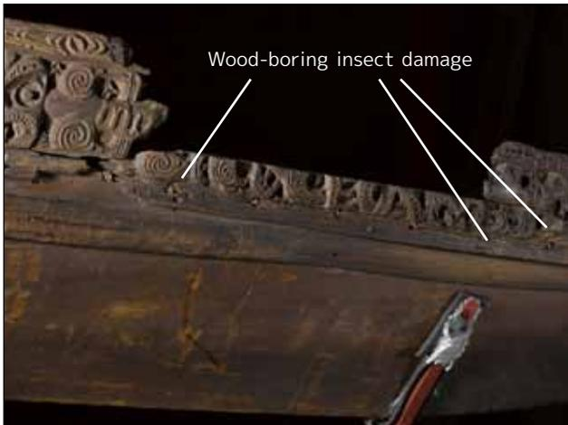
**Fig. 7:** Detail showing incomplete starboard *Rauawa* and *Taka* nailed to hull, with insect damage.
