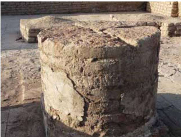
**Fig. 13:** Brick and lime rendered column, 2011.
