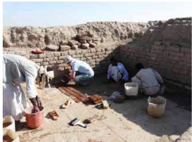
**Fig. 5:** Bedding the brick infill.
