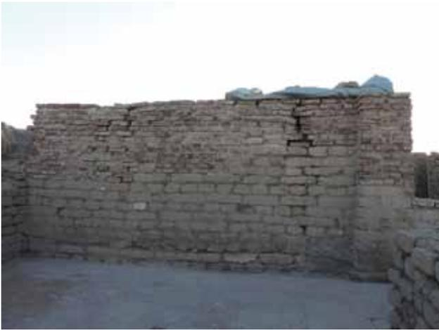
**Fig. 11:** Failed pointing to capped wall.
