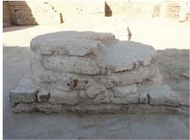
**Fig. 12:** Failed lime render to brick column.
