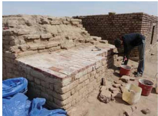
**Fig. 9:** Finished capped wall
