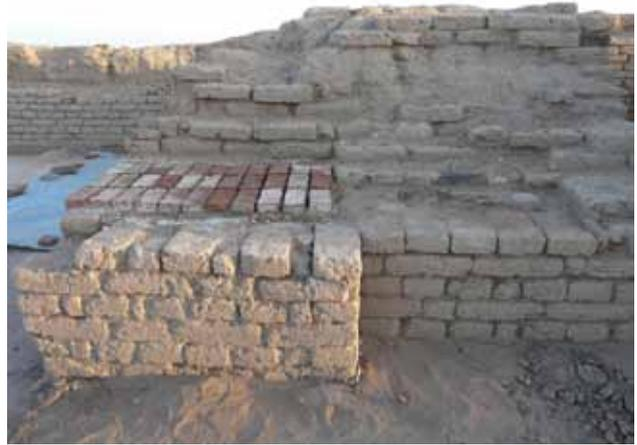
**Fig. 8:** Capping exposed walls
